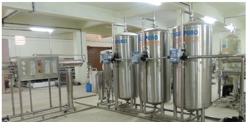
Aguapuro Water Softeners use the proven technique of co-flow and counter current regeneration. Co-flow operates with regeneration flow in the same direction as service flow, and counter current involves the flow of brine used for regeneration and the flow of raw water during service, in opposite directions to each other. This ensures the residual hardness in treated water is always less than 5 ppm as  $\text{CaCO}_3$  throughout the cycle.
